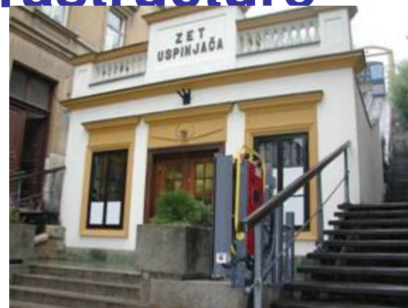
Adjusting old building, Zagreb
